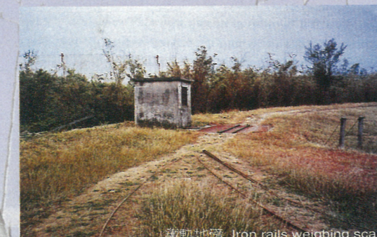
鐵軌地磅 Iron rails weighing scale
