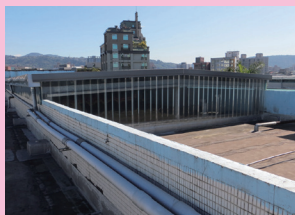
斜屋頂隔熱防漏
